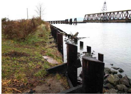
Figure 8. Creosoted treated timber bulkhead
