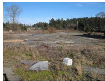
Skagit Plastics factory foundation
