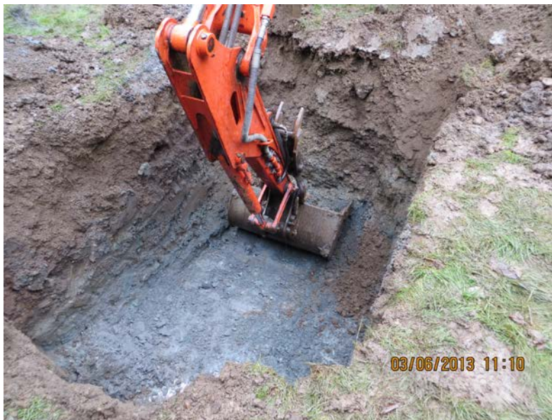
Abandoned heating oil tank remediation (Kukutali Residence)
